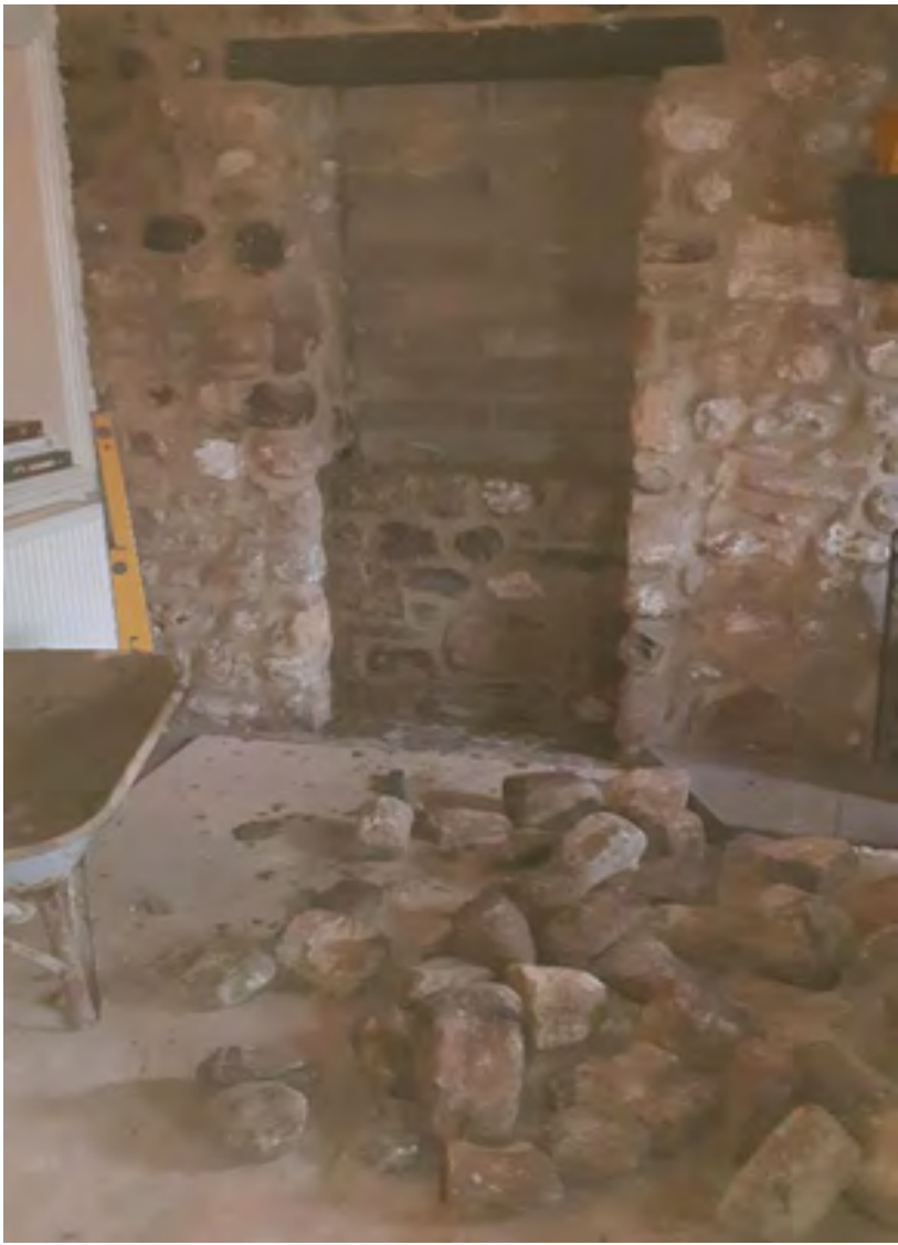
Within the rubble that came out of the knock through were a load of cobbles. These were recycled to form a wall to the left of the main pub fireplace to block off the old access to the pub toilets - so a bit of history from the property has been retained and reused.
